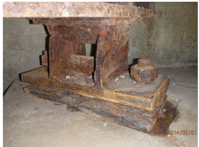
Existing steel bearing
