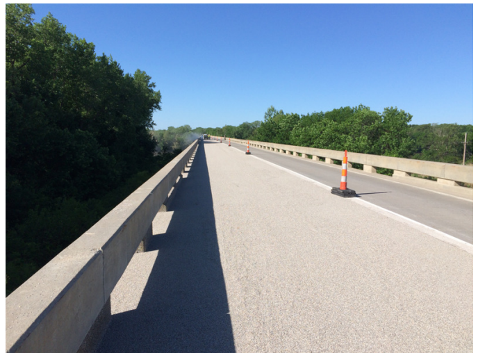
Overlay Route 1029 Kansas River Bridge completed 2017
