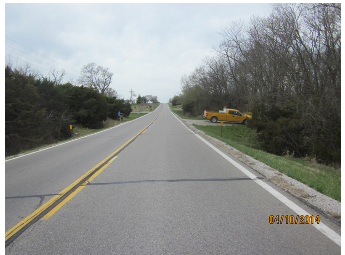
Existing shoulder condition
