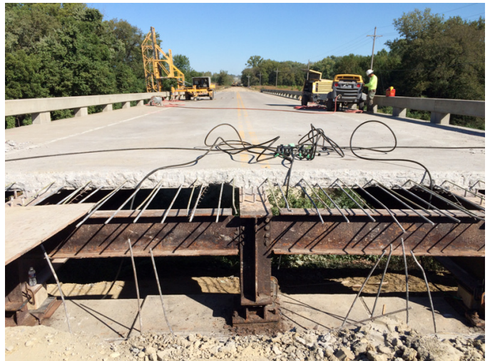
Repair work on bridge 1186-1500
