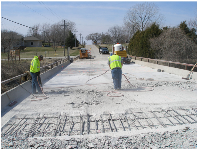
Concrete deck repairs
