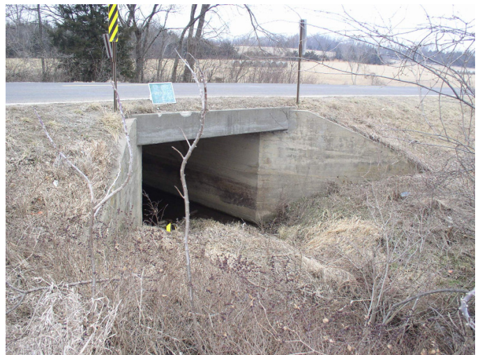
Existing narrow culvert
