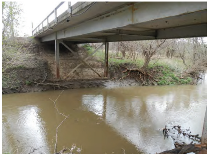
Existing steel girders
