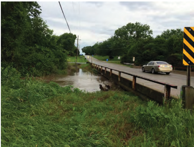
High flow at bridge 1100-1330
