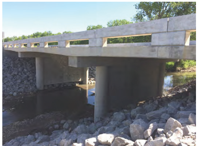
Replacement completed May 2017
