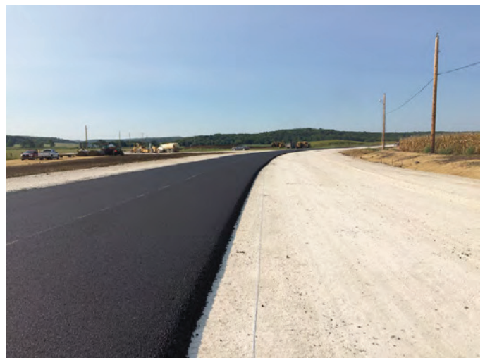
Three existing 40 mph curves have been realigned
