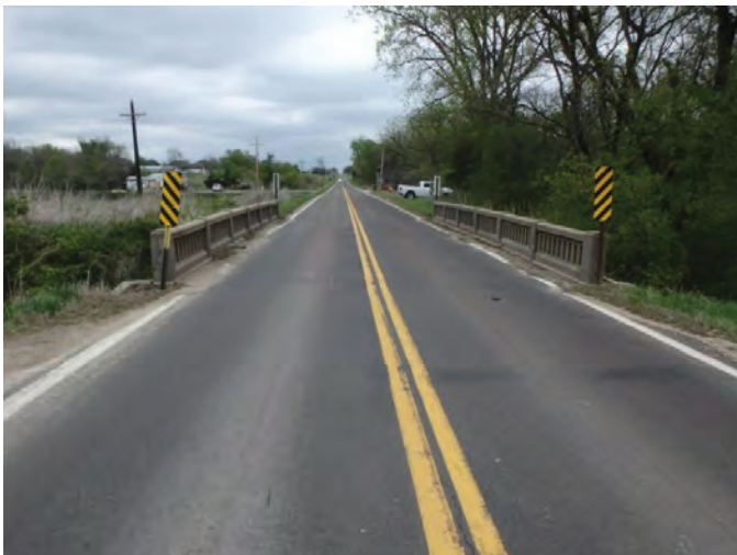
Roadway before replacement
