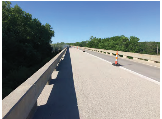
Overlay Route 1029 Kansas River Bridge completed 2017
