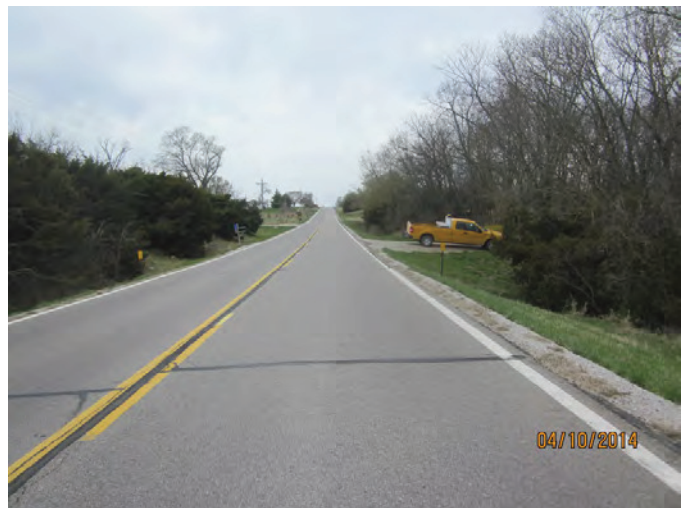
Existing shoulder condition
