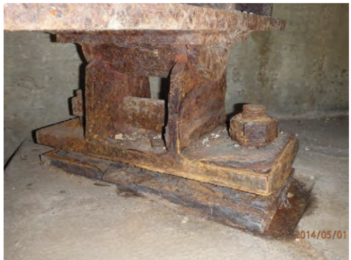
Existing steel bearing
