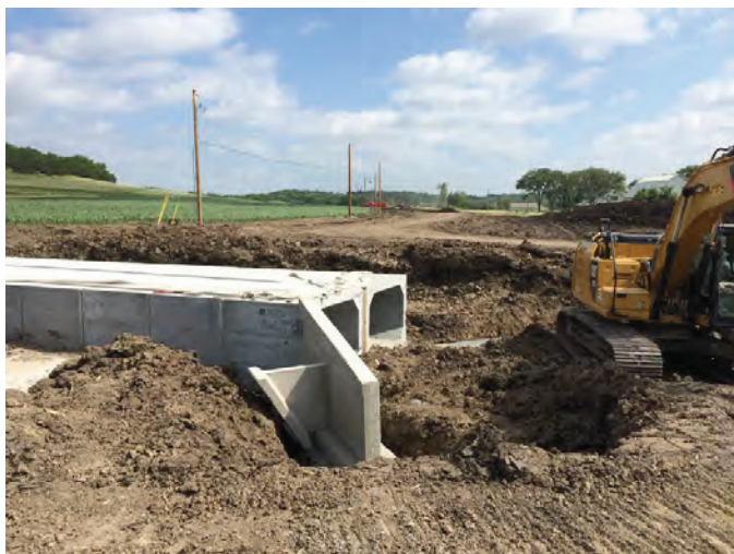
This project includes 28 new road crossing culverts
