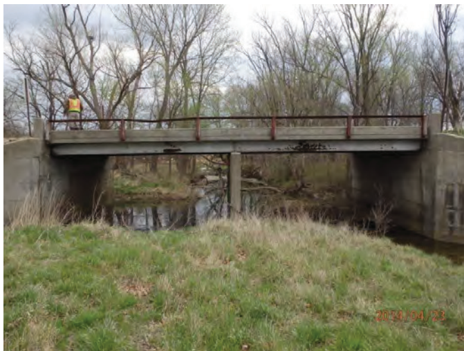
Existing bridge in 2016
