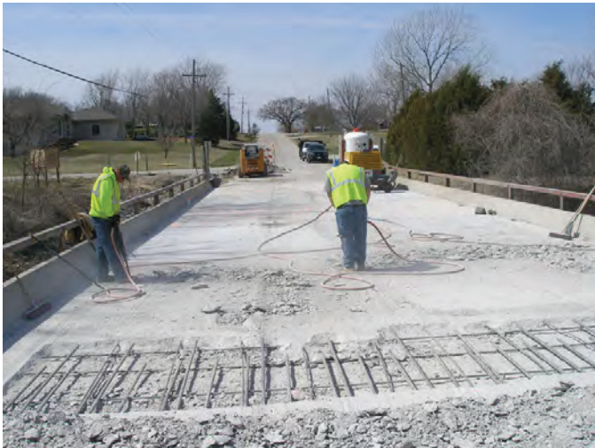
Concrete deck repairs
