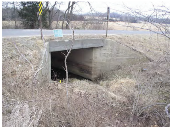
Existing narrow culvert
