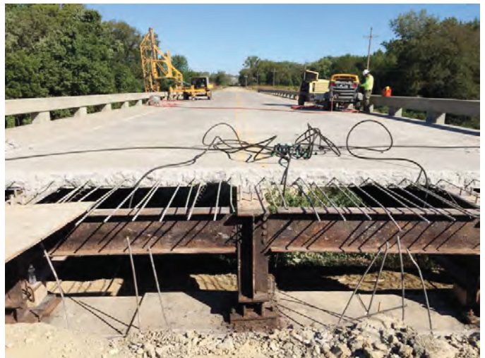
Repair work on bridge 1186-1500
