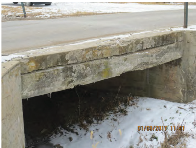
Existing narrow culvert on N 1500 RD (E 15th St)
