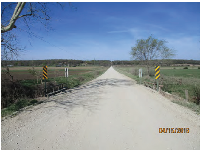
Existing narrow culvert
