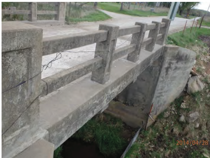
Bridge prior to replacement
