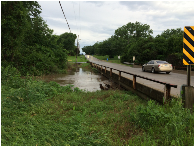
High flow at bridge 1100-1330
