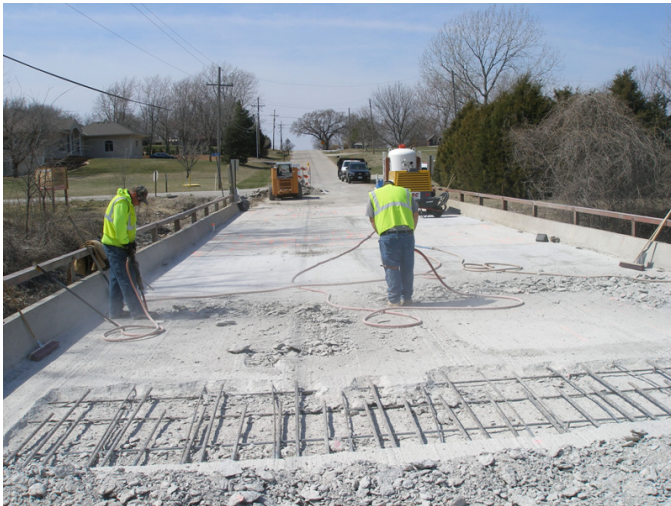
Concrete deck repairs
