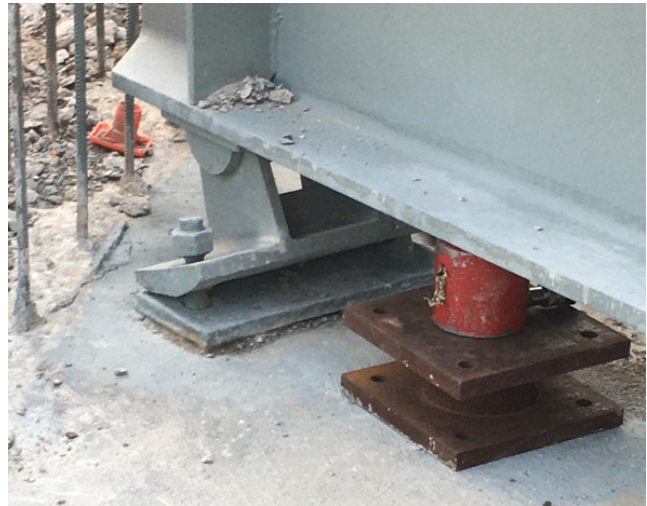
Replacement bearing installation
