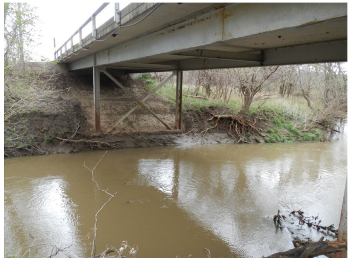
Existing steel girders
