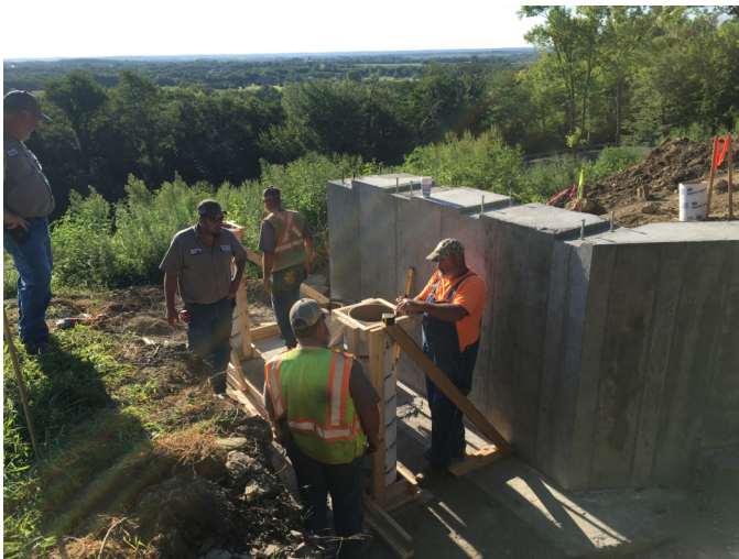
Foundation construction by Public Works crews
