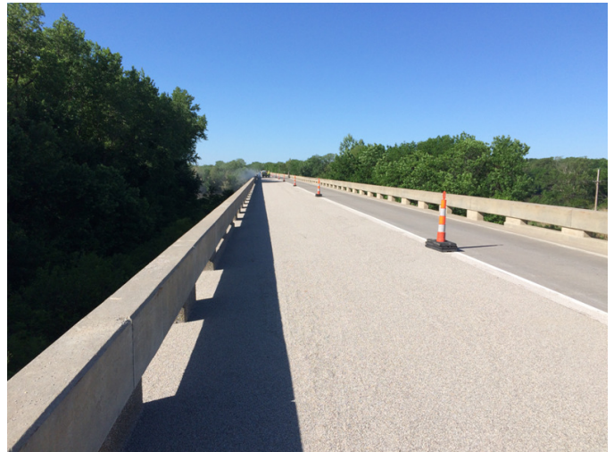
Overlay Route 1029 Kansas River Bridge completed 2017
