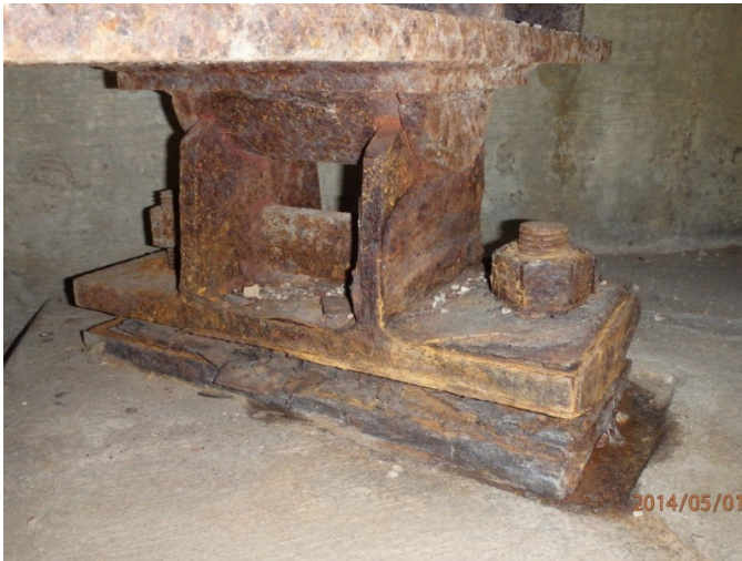
Existing steel rocker bearing
