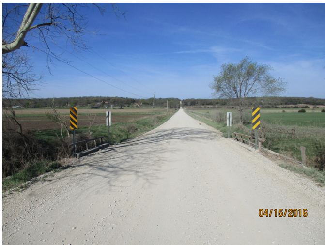
Existing narrow culvert
