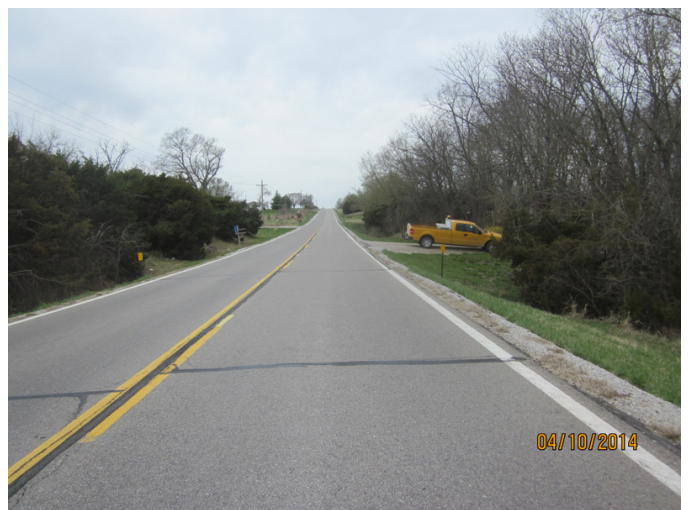
Existing shoulder condition
