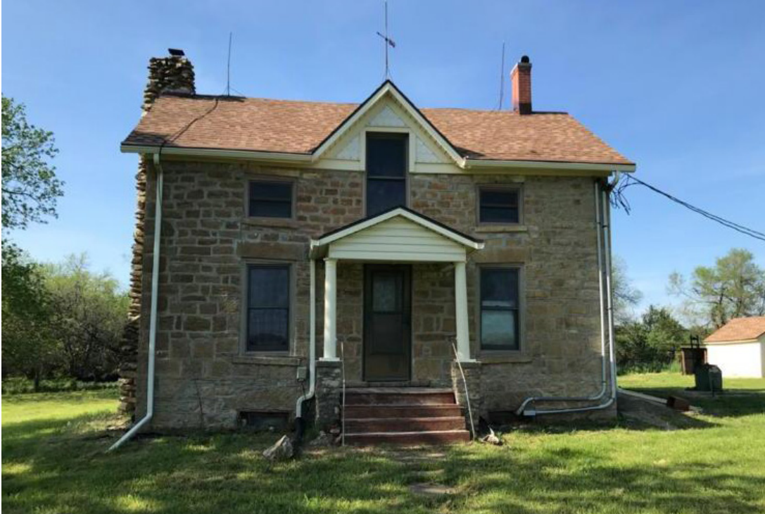
The McQuillion House was built as early as 1856 when Thomas McQuillion first settled in Willow Springs Township. The centered gable, reminiscent of vernacular Gothic Revival houses, was likely added in ca. 1870. Photo by Christy Davis.
