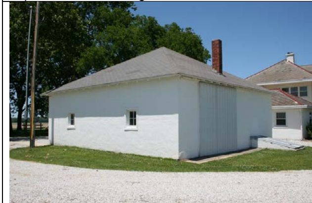
Shed, Granary, Potato Cellar – 1359 N 1900 Rd
