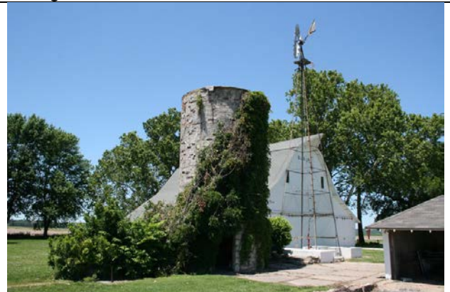
Water Tank & Windmill – 1359 N 1900 Rd
