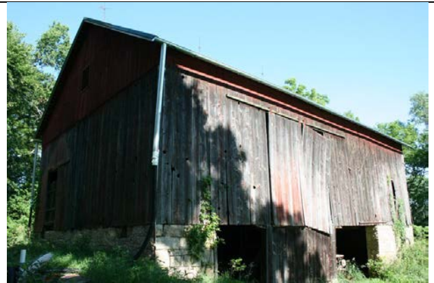
Anderson Barn – 1862 N 700 Rd
