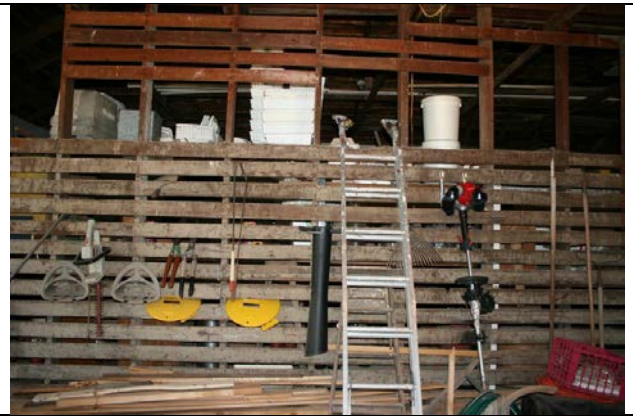
Corn Crib & Shed - 1359 N 1900 Rd
